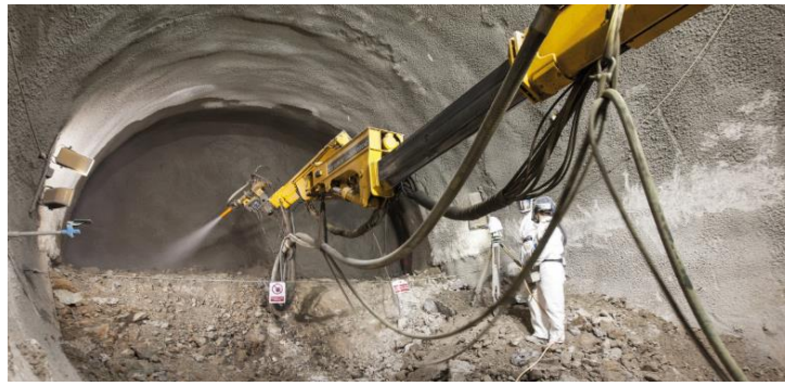
Figure 11. Fiber-Reinforced Shotcrete Surface
