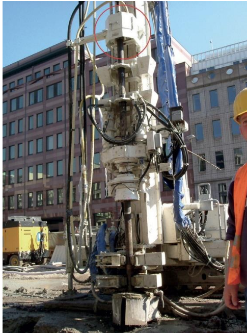
Figure 6. Jet Grouting Drilling Stage
